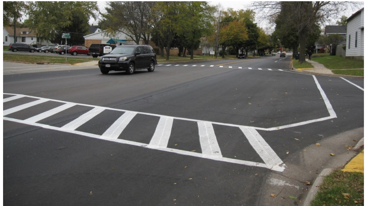
The Fort Atkinson Public Works Department oversees projects along City streets, such as these high-visibility crosswalks near Barrie Park.
